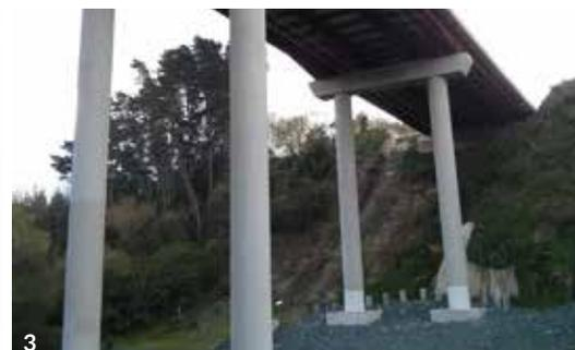
1 Horotiu Paa Bridge Cambridge Pier Connection 2 Horotiu Paa Bridge Cambridge Weathering Steel 3 Horotiu Paa Bridge Cambridge Columns Scour Protection and Shear Piles
