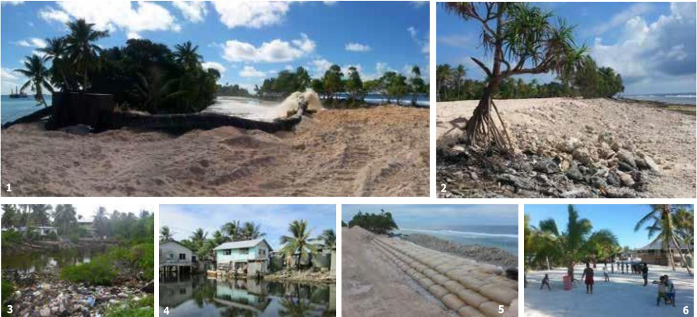
**1** Action shot of the dredge pumping through the bomb box and into borrow pit (Tom Henderson) **2** Completed breach repair (Tom Henderson) **3 & 4** Borrow pits 4 and 7 before remediation (Peter Ollivier) **5** Breach repair (Tom Henderson) **6** Communal activity in Borrow pit 7 after remediation
